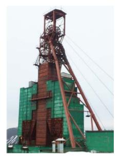
The single-layer double drum with a diameter of 5 m lifts a load to a height of 480 m in around 11m/s. After 244,000 cycles, the rope was removed, and the areas exposed to the greatest stress during operation in the mine were examined in the lab. Neither the loss of profile nor the wear and corrosion on the inner side of the rope were significant as yet. The breaking strength measured was, despite the high number of load cycles, still above the minimum breaking strength guaranteed at delivery.
